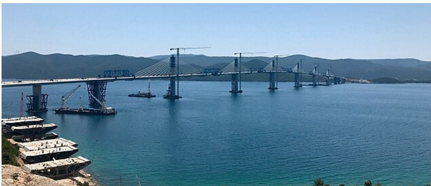
Figure 4. Pelješac bridge under construction. Source:Ponor / Wikimedia Commons (CC BY-SA 4.0)
