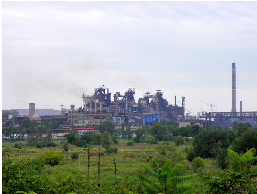
Azovstal iron and steel works in 2021 (27 August 2021). Photograph by Blast furnace chip worker, licensed under CC BY-SA 3.0, via Wikimedia Commons. Available at: https://commons.wikimedia.org/wiki/File:Azovstal_iron_and_steel_works_in_2021
